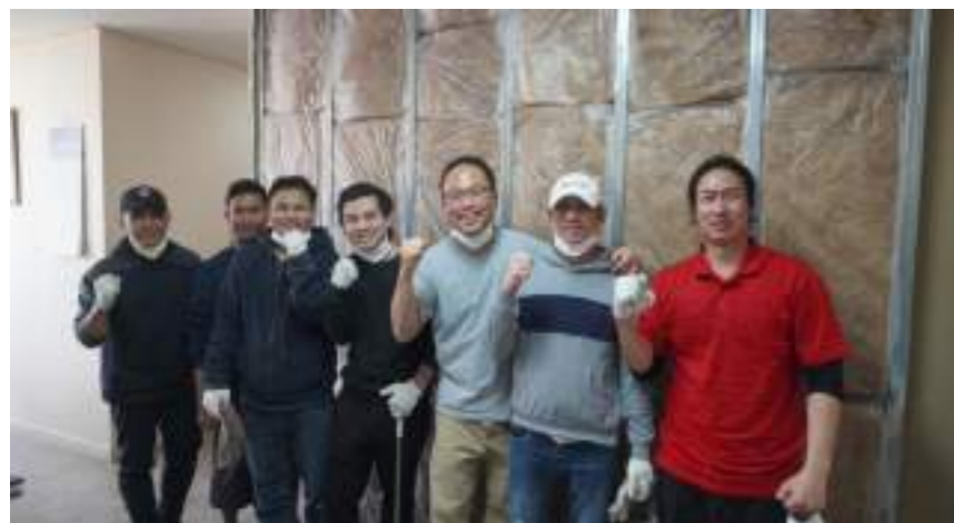
With shelter residents during shelter repair work
