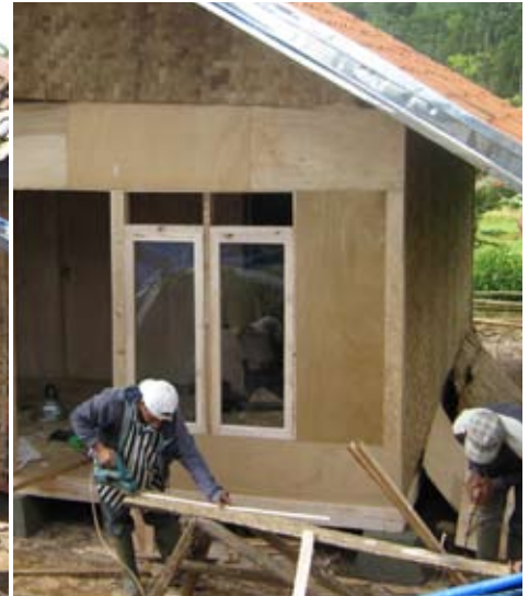
Construction workers in Bungbangsari Village.
